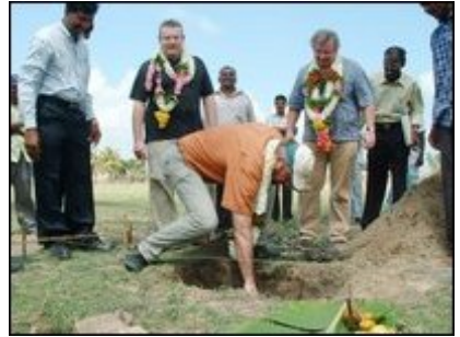
Mr.Meinoff Schwefer laying foundation stone for the two storied pre-school in Veloor
